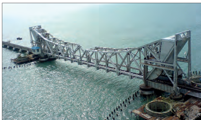
Fig. 7: Pamban Rail Bridge (Photo: Wikipedia)
