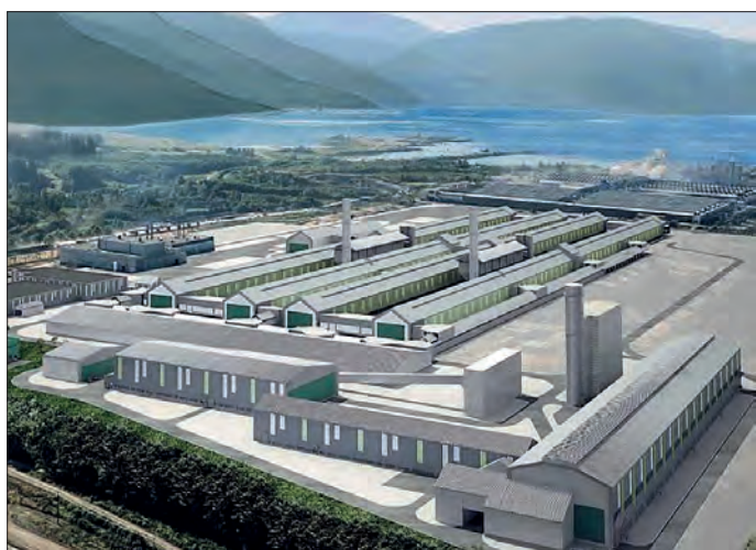
Fig. 2: Kitimat aluminium smelter is one of BC's largest manu- facturing complexes
