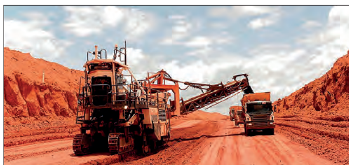
Fig. 1: Clearing up the existing stockpiles of bauxite in Kuantan has proved a harder task than anticipated (Photo: Norsk Hydro ASA)
